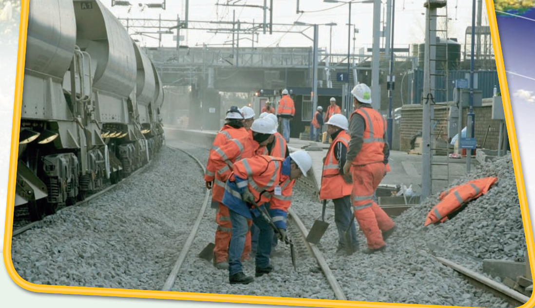
Train rails can buckle in hot weather, so trains need to go more slowly in hot climates.
